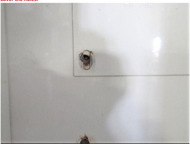
When holes are lined up, install 7 freezer screws (RA), if you are wanting to use new screws use a 2" X #10 screw, pull the unit tight against the back. If holes do not line up exactly you can easily angle the screw up/down side/side to get to the hole as these holes are set in approx. 1" from the front of the foam pack.
