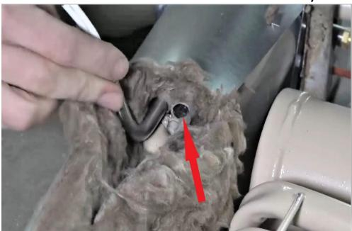
Lay the unit on its back and place a small bead of thermal mastic as shown in red. You will need to use the the entire tube.
