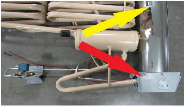
Open the heater cover and push the insulation back so the heating element sockets are exposed, and slide the heating element into the socket. It does not matter which socket you choose. Make sure it's pushed all the way down to the stop point on the heating element. Push insulation back over the heaters and install the cover and tuck the heater wires out of the way for now.
