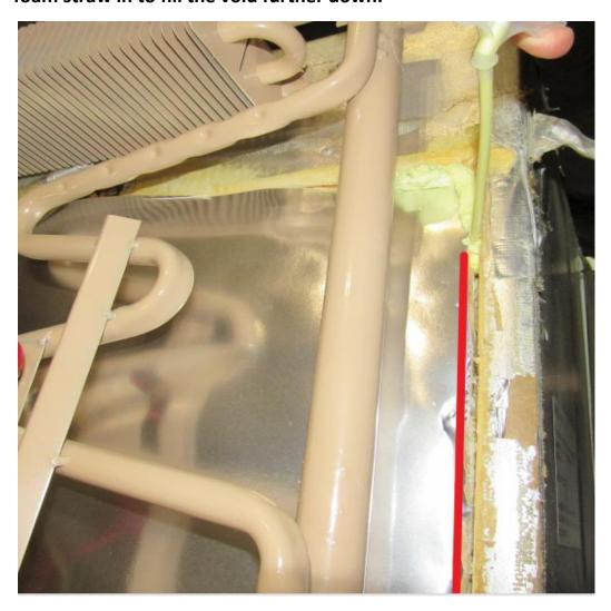
After filling the gaps with foam, follow up with the supplied aluminum foil tape on all 4 sides. This foil tape is for cosmetic purposes only, it does not help the seal between unit and box.
