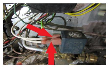
Plug in the black 120V cord into the bottom left corner (RA) of the board, plug in the 2 fan wires, (GA) make sure the black is on the right & white on the left. Plug gas valve wires back into board spades marked GV & GV GND (YA) Plug igniter wire back in (RA)
