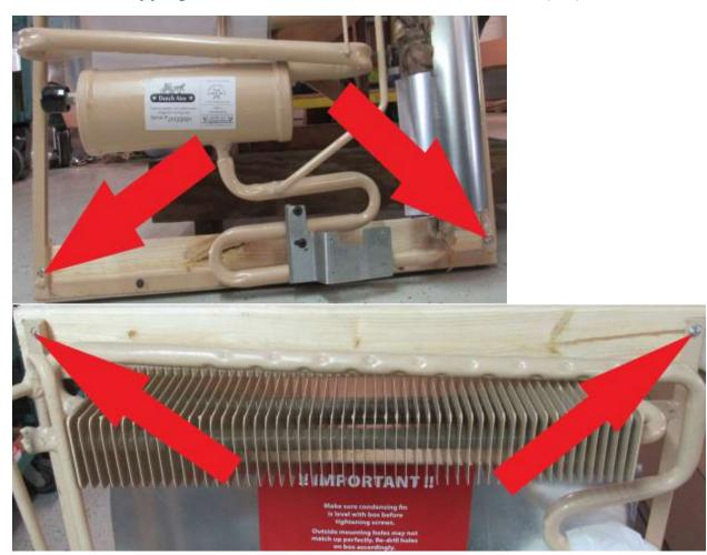
The steel brace does not need to be removed (BA)
