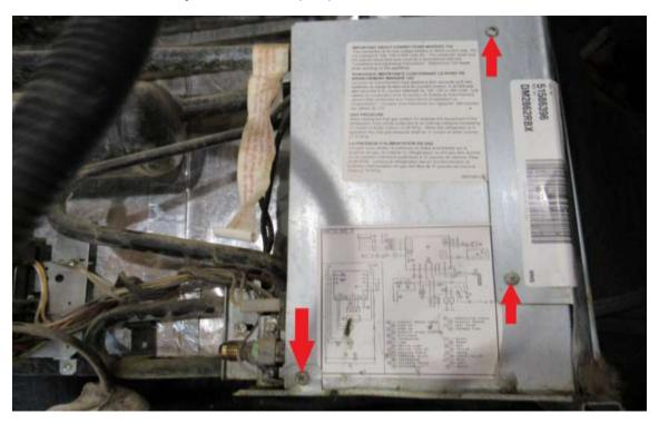
Remove the high temperature switch screws (RA). Sometimes this switch is pop riveted in place, so removing it by drilling the pop rivet heads off is the easiest option.
