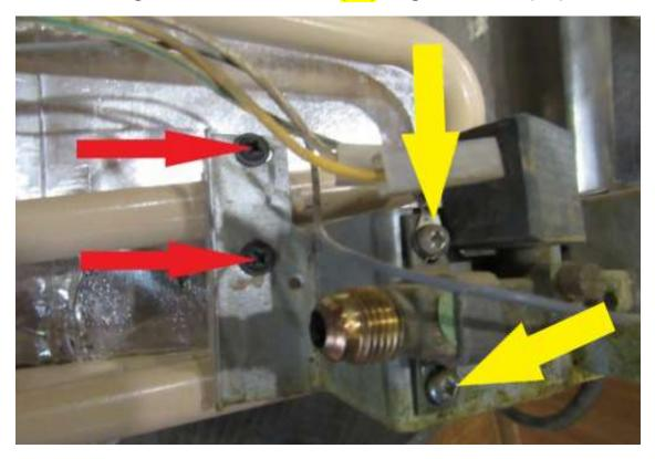
Install the high temperature switch as shown using the original screws (RA). If you do not have screws then use only very short screws to attach to the insulation pack only, do not drill or run a screw into the boiler tube itself
