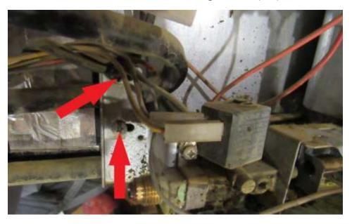
You will now be able to completely remove the control board and burner assembly and it should look like the picture below.
