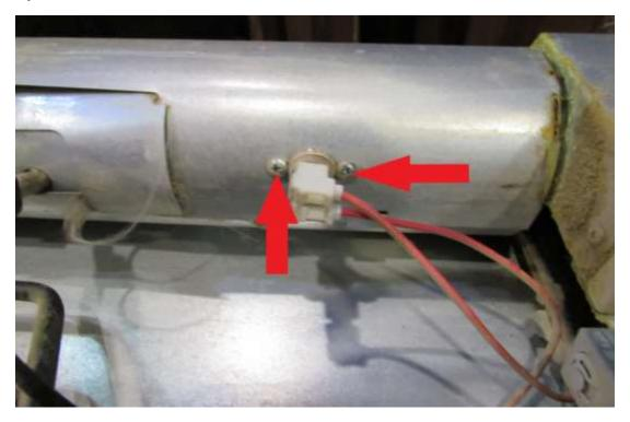
Next, remove the burner cover (RA). If you have yellow residue from a leaking unit, it should be cleaned before re-installing. Plain water clean up
