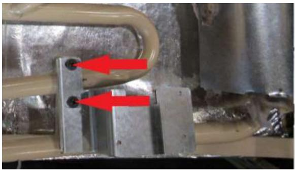
Slide the burner assembly on top of the flue bracket and install the burner set screw RA).
