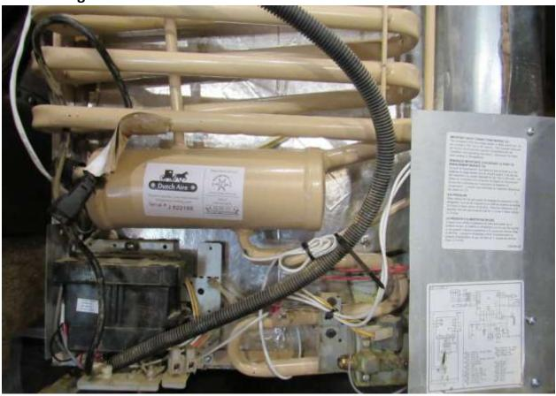
Before installing the fridge back into the cavity, check to make sure wall insulation is secured and this is a good time to sweep or vacuum any loose debris. If this fridge is installed into a slide out then make sure and remove the top side vent (YA) baffling (RA), as you will no longer need this and all it will do is slow air flow.
