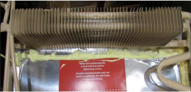
After filling the gaps with foam, follow up with the supplied aluminum foil tape as shown. This foil tape is for cosmetic purposes only, it does not help the seal between unit and box.
