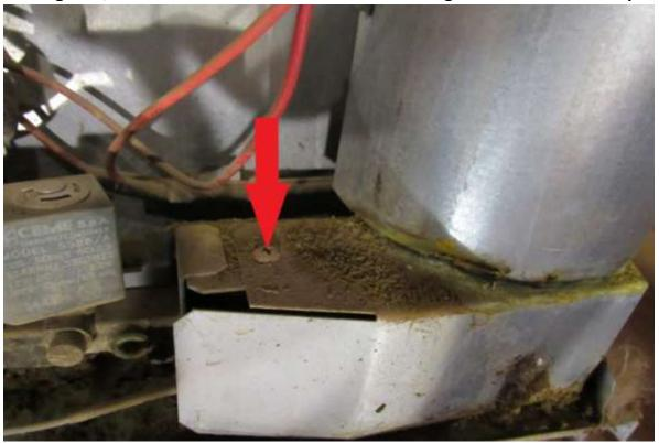
Remove the burner set screw (RA).
