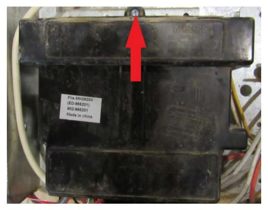
Slide the burner cover into place and fasten into place with the original screw (RA).
