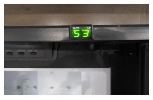
Now plug your 120V plug back into the wall outlet and make sure you have 120V AC power to this outlet. LP burner should now shut down and board should switch to AC. If you have a amp clamp the total amps on the heaters should be 3.6A to 3.8A. After its been running for ½ to 1 hr you need to make sure you here the rear vent fans turn on. Which can be heard either thru the front fridge door or thru the rear side vent
