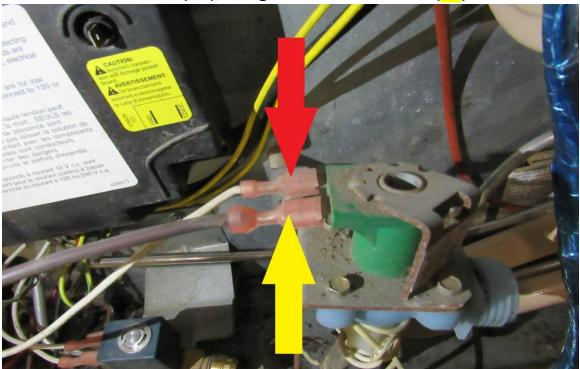
Connect the ice maker hose to the solenoid (RA).
