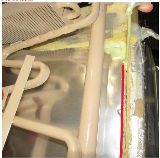
After filling all gaps with foam, follow up with covering the edges with the supplied aluminum tape. This does not serve as a seal but for cosmetic purposes only.
