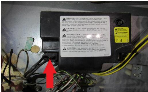
Plug the igniter into the board (RA) as shown.
