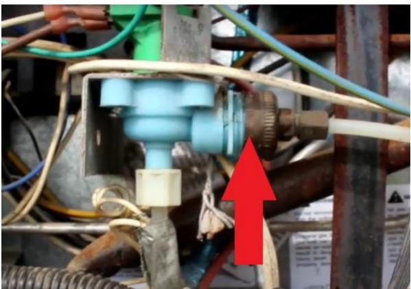
Using 2 wrenches remove the LP line (RA) off of the LP solenoid valve. Make sure LP gas is turned off.
