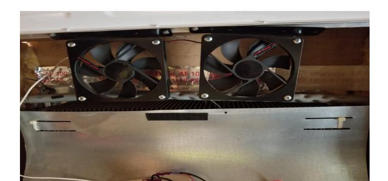
You will then be required to add a slideout fan to your top side vent to force the hot air out that's being pushed up from the fans below the vent, (this is required on all slide out models to be covered in our warranty)
