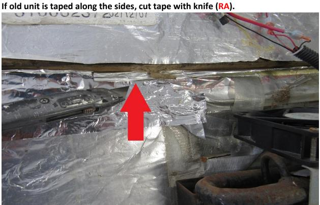
Take off the old cooling unit of your refrigerator by lifting straight up and out. We will need to take some parts off of the old unit later. Clean off any residual foam or thermal sealant around the edges (RA).
