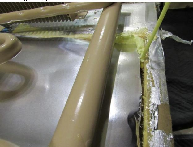
In some areas it might seem to be tight against the box, and in this area cut back enough foam on a angle to create a small gap off the unit so you can get your foam straw in to fill the void further down. We cannot stress enough on this step because if even a small 2" gap is left open it will not cool in the fridge like it should.
