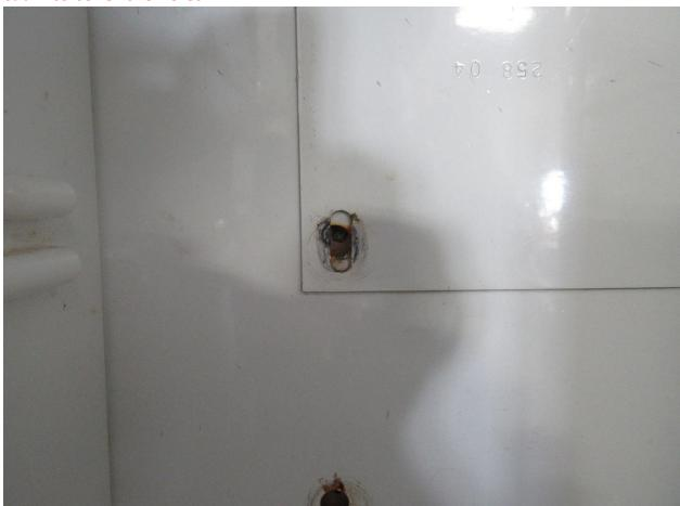
When holes are lined up, install 8 freezer screws (RA), using the supplied screws in the parts bag, pulling the unit tight against the back. Do the same with the refrigerator section fin (RA). Install seven screws pulling it tight.
